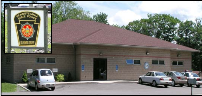
State Police Barracks, Route 402
