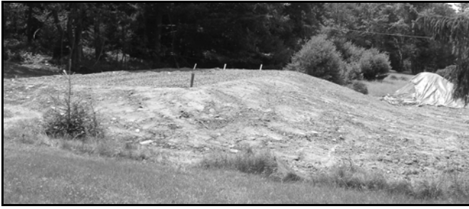
Sand Mound Under Construction
