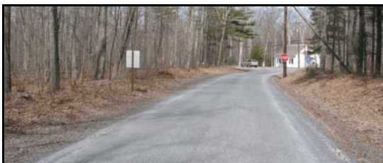
Snow Hill Road - Township Road 317
