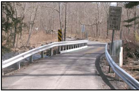
Bushkill Creek Bridge - Snow Hill Road
